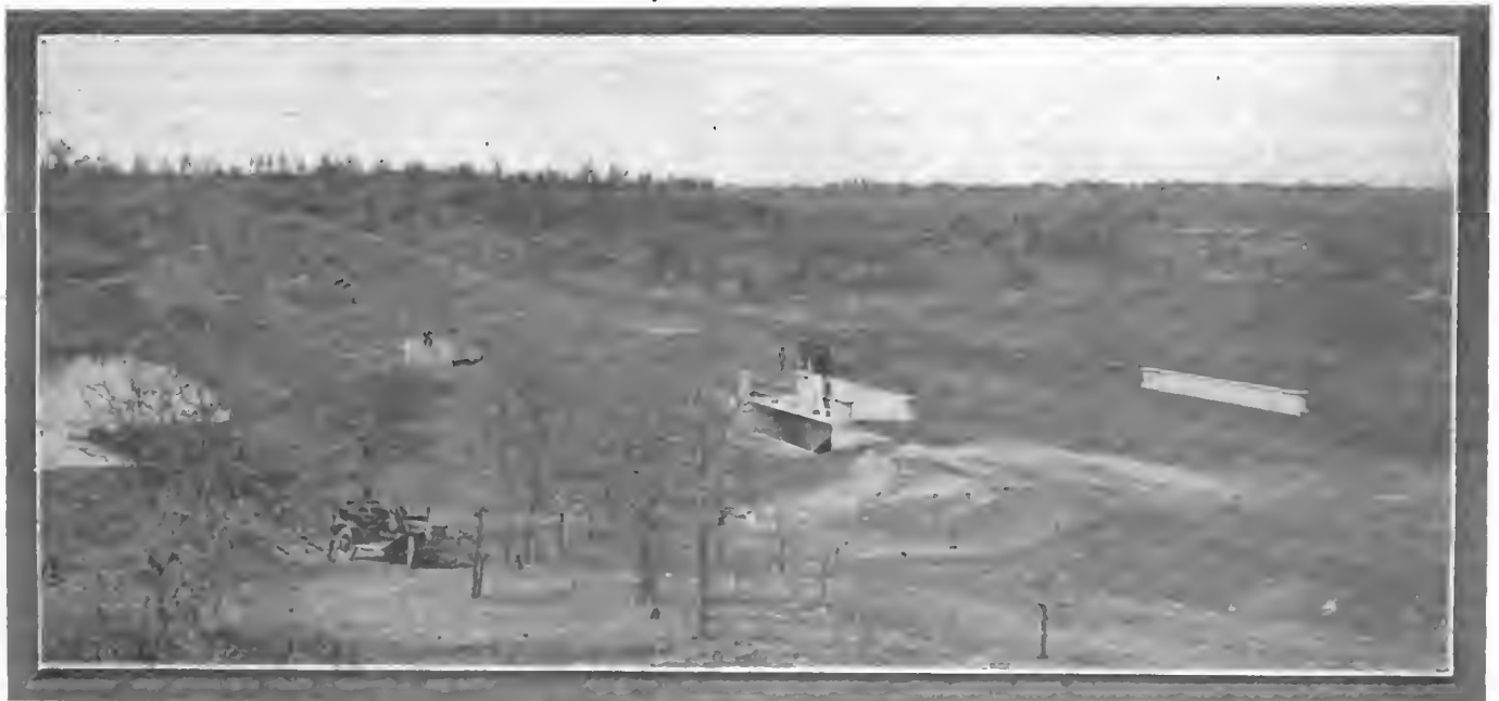
View of the 26-mile automobile speedway at Oklahoma City. All grade crossings have been eliminated and one 3 per cent. incline is the steepest
